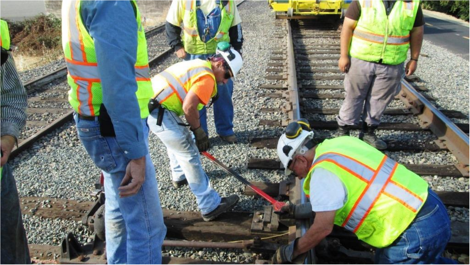
Joe and Clem loosen the bolts on the wedge-bracket at Switch 13
