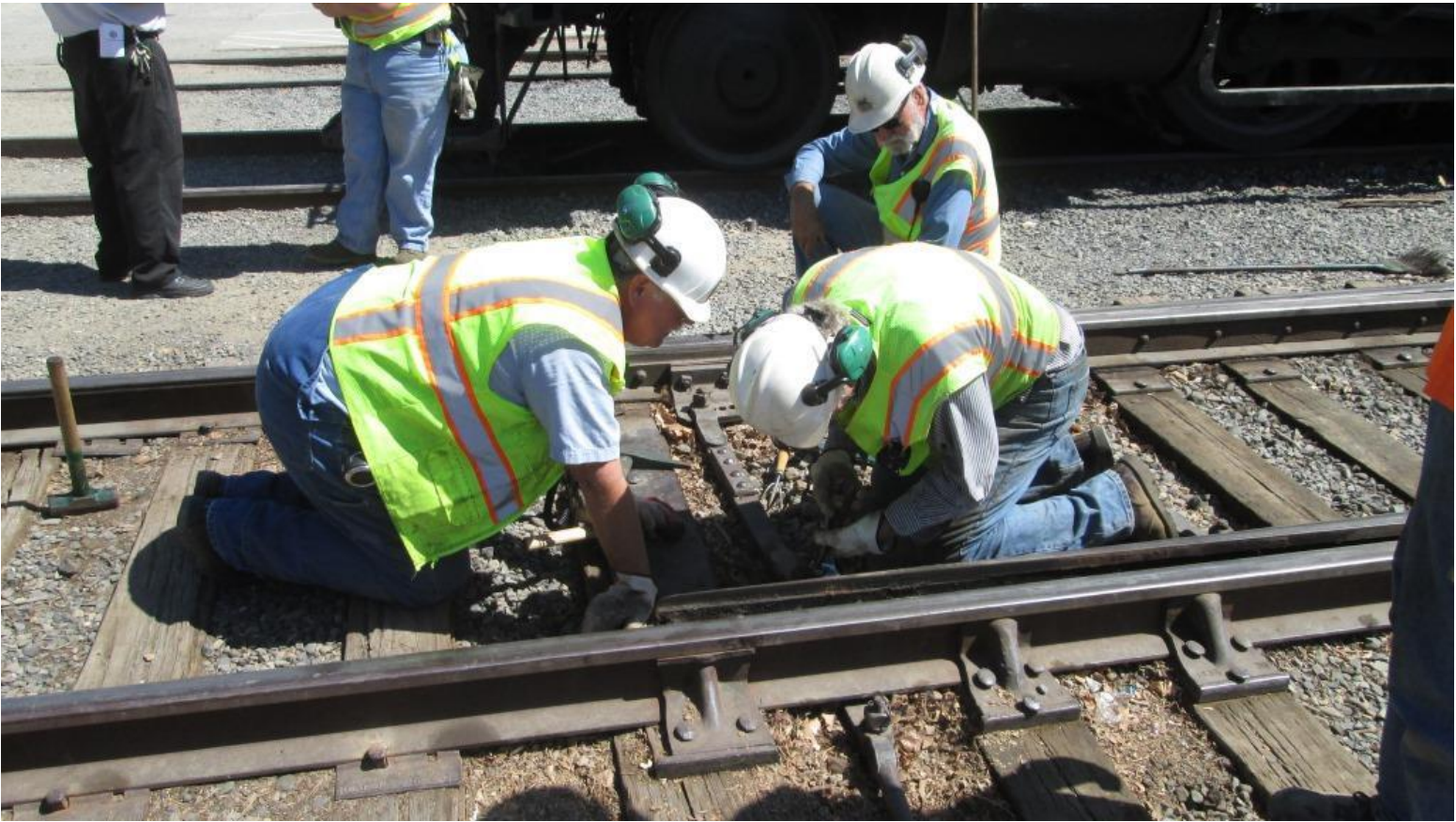
Chris and Steve replace the bolt holding the connecting-rod in place
