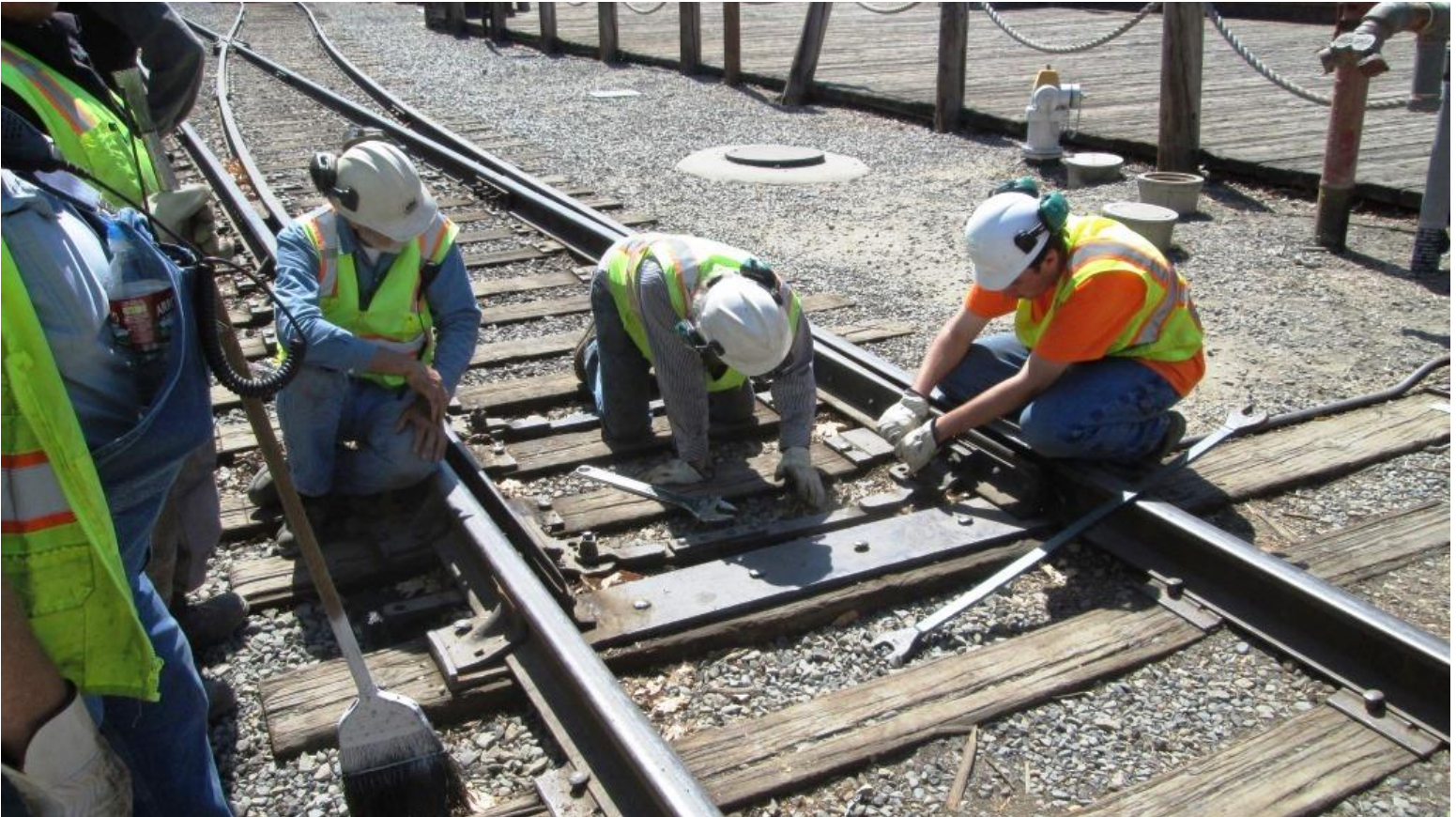
Now on to Switch 8 where Steve and Weston remove the connecting-rod bolt to the transit-clip
