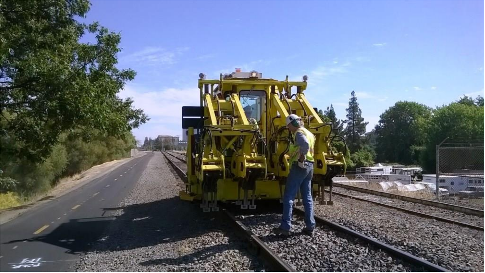
Now Heather's crew tamps near the switch
