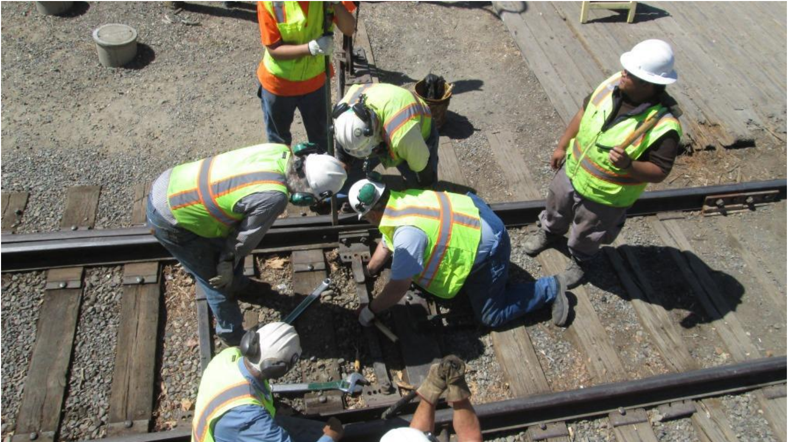
Chris, Steve, and Mike F. adjust the position of the connecting-rod on the transit-clip
