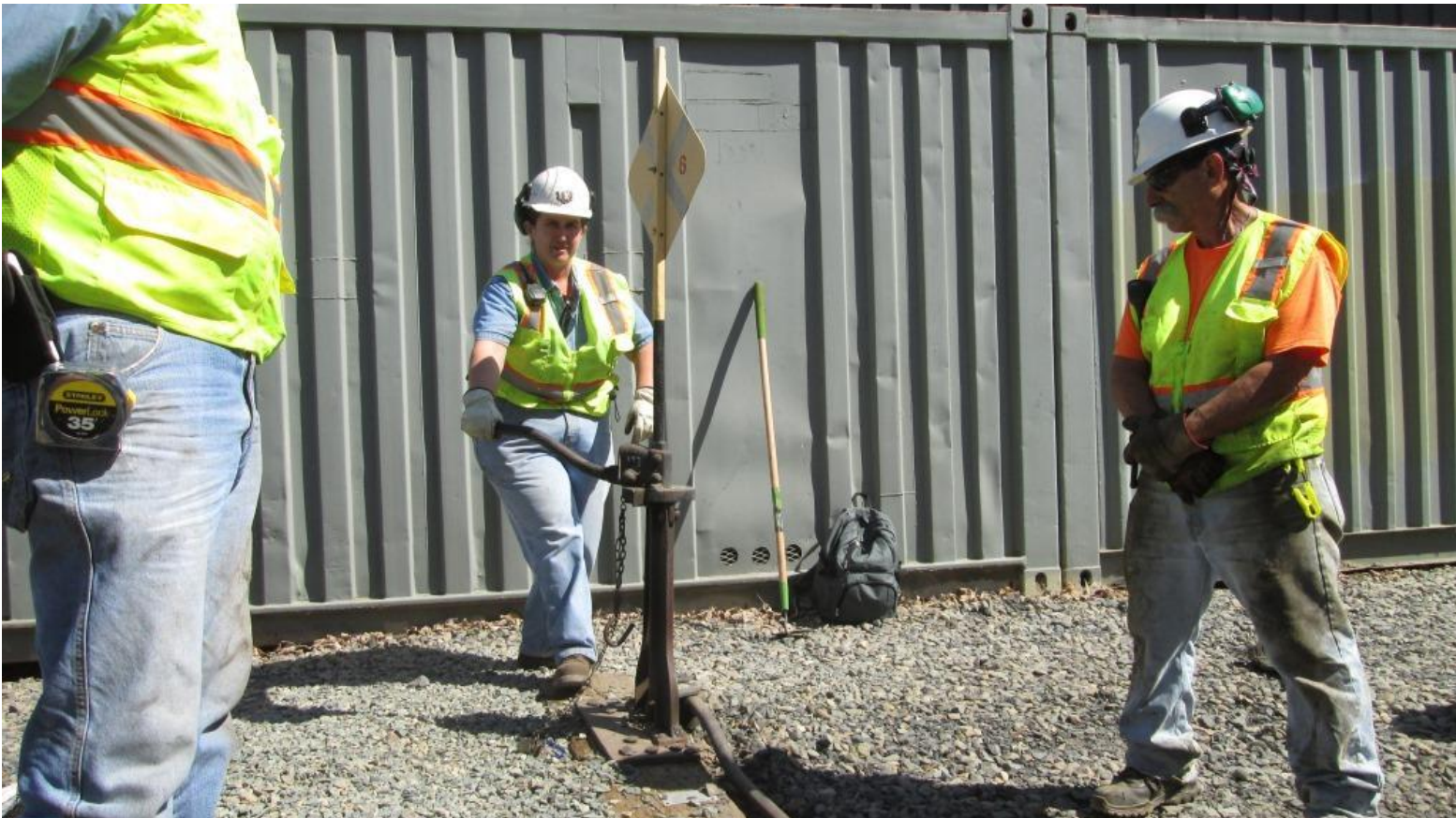
With all adjustments made, Heather now throws Switch 6 with one hand
