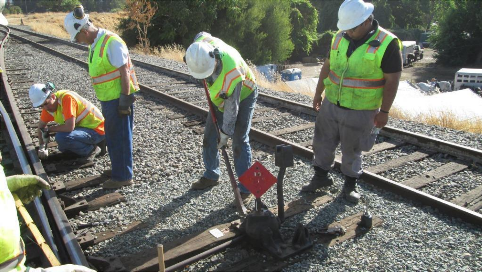
Steve pulls spikes on the switch machine
