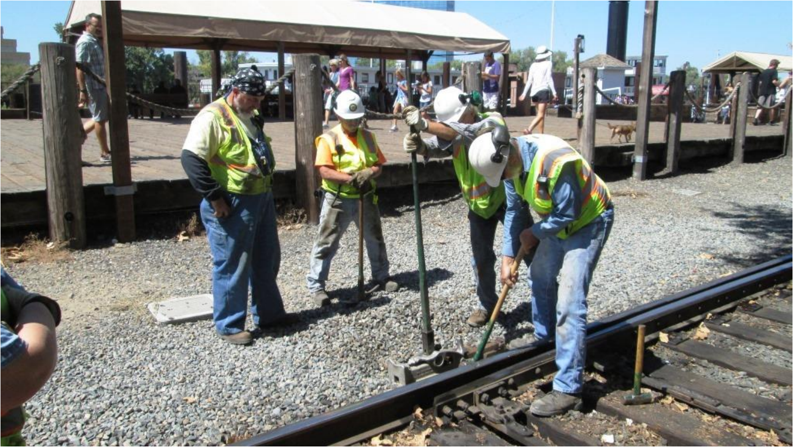
Steve cranks on the jack as Alan give the tie a few whacks to shimmy it over a few inches
