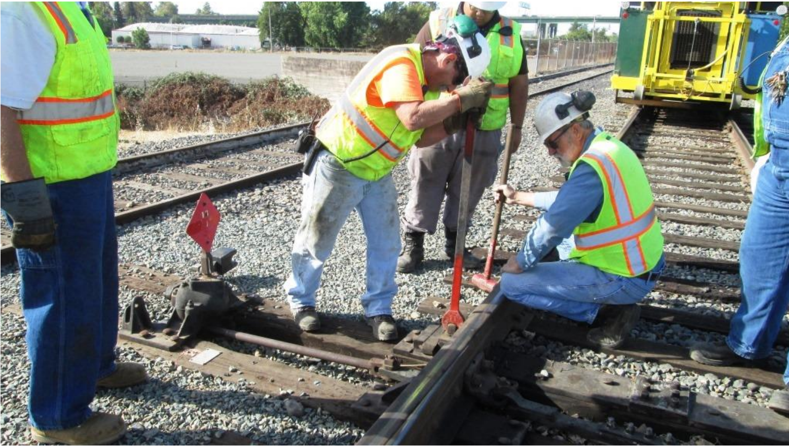
Joe tightens-down the bracket-bolt
