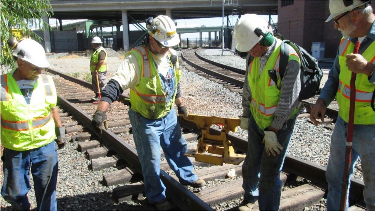
Mike F. and Steve move the derail device to a more secure location
