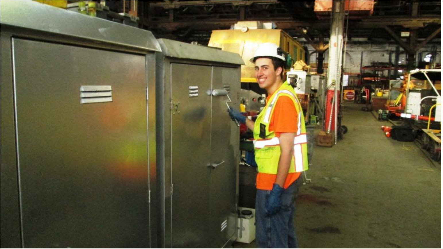
Paint, paint here, roll, roll there and a couple of tra-la-las. That's how we work the day away in the merry ol' land of MOW...
