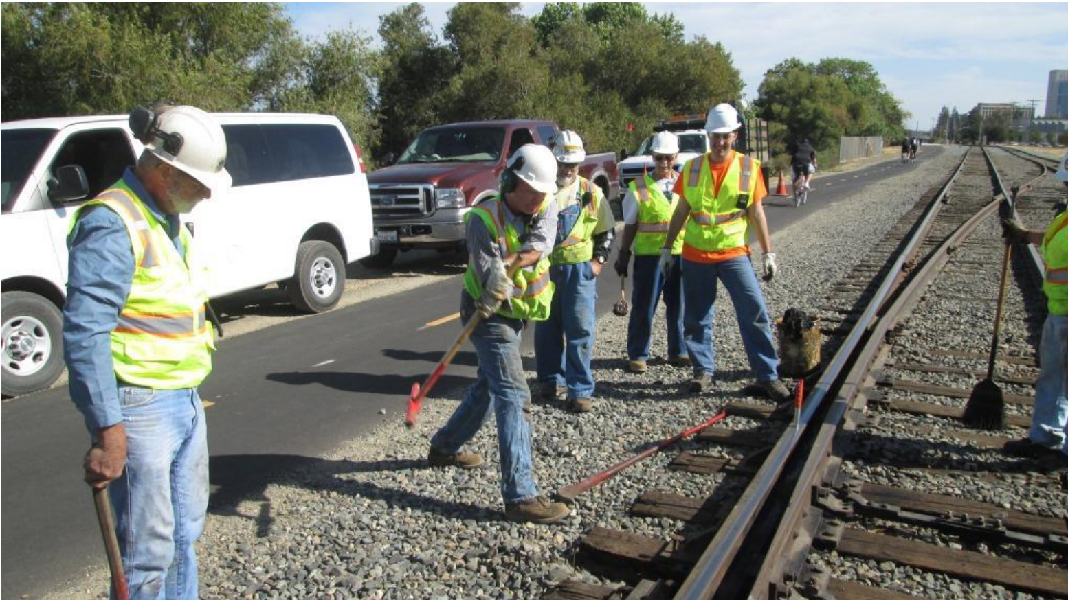
Steve demonstrates his world-famous as-seen-on-TV windmill spike-driving technique
