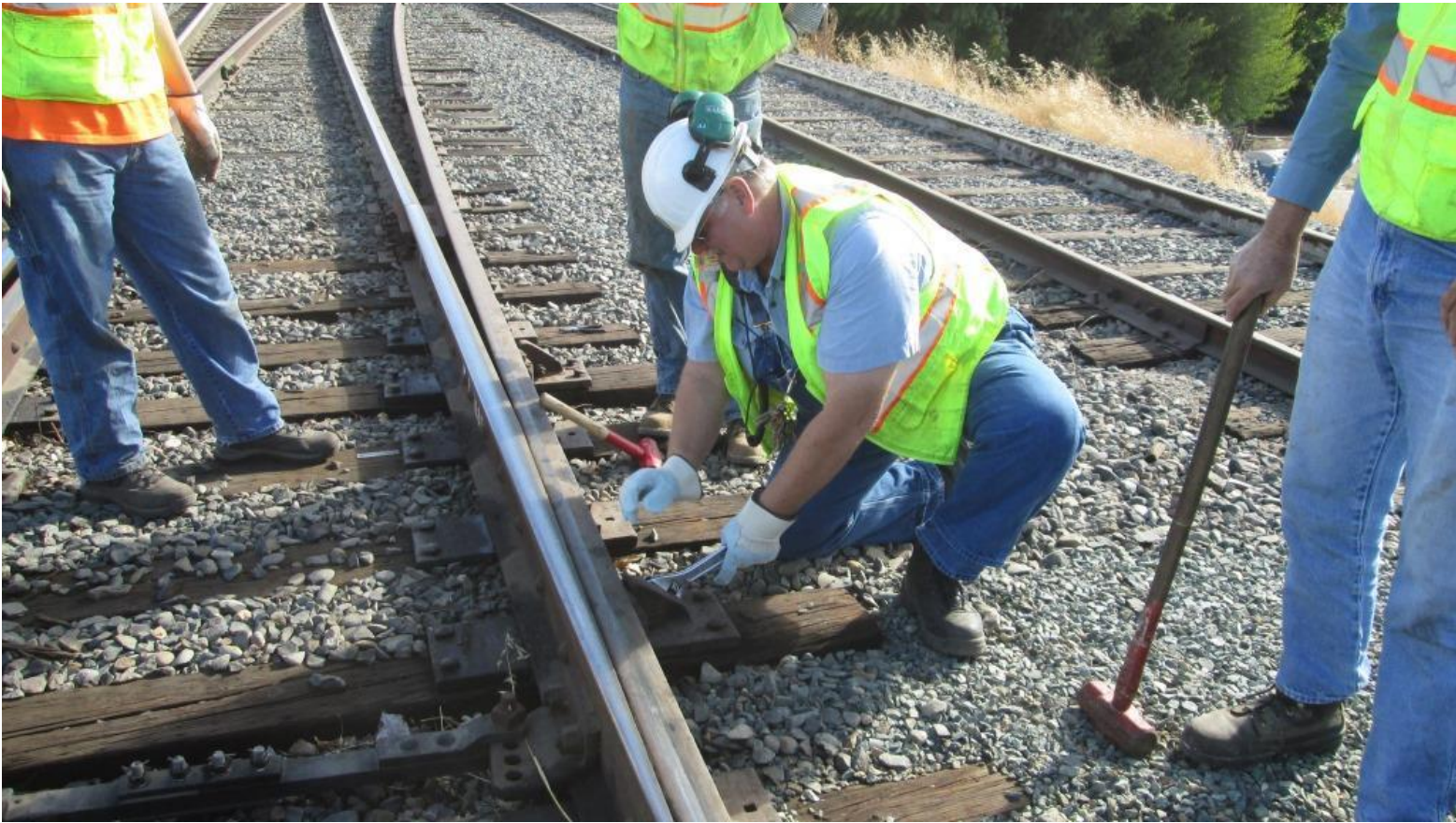
Chris removes the "keepers" on the bracket at Switch 13
